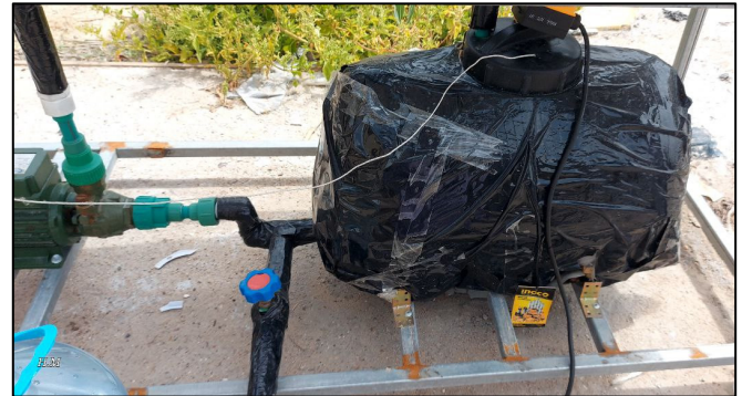
Fig. 3 The photograph of the saline water reservoir.
