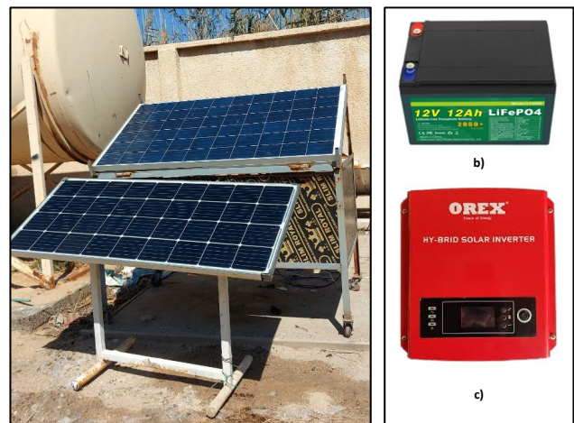
Fig. 4 PV panel component (a) photovoltaic cells, (b) lithium iron phosphate battery, and (c) hybrid solar inverter OREX.
